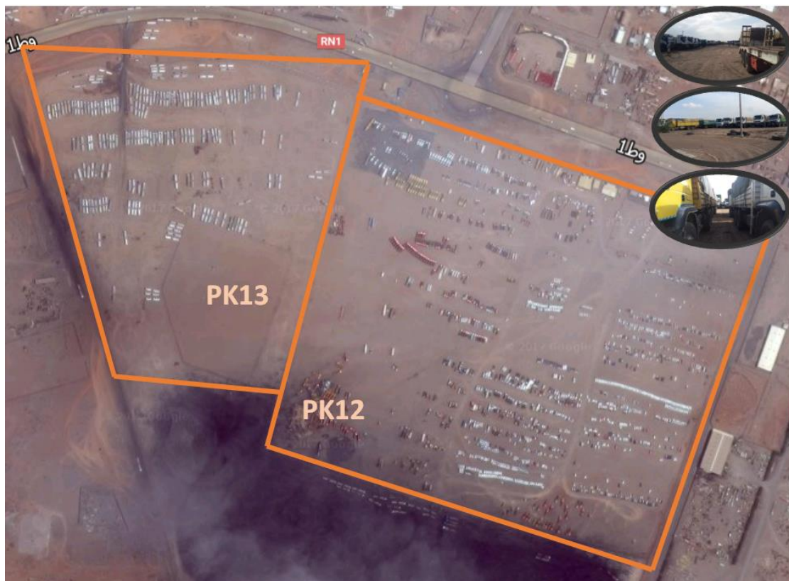
Figure 3 – Infrastructure – Truck Park and Holding Area
